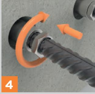
Screw the coupler by hand onto the 1st phase rebar. A wrench may be used to ease operation.
