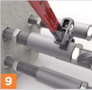
Use a wrench to tighten the couplers onto their matching rebar.
