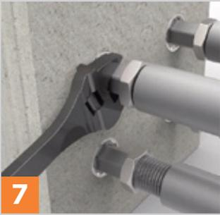
Rotate each stud with a wrench to find the correct engagement position.
