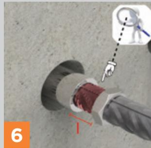
Check the distance "l" between the coupler and lock nut (still engaged at the bottom of the long thread) it has to fall between the limits indicated in table 5 below.
