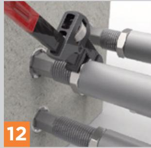
Tighten the lock nuts with a wrench.
